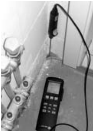
Abb. 7: Messung in Estrich-Randfuge
